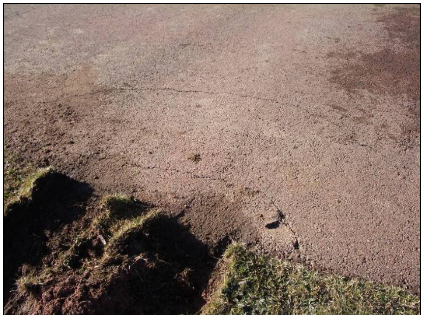
Photo 2. Runway edge damage from right main landing gear
