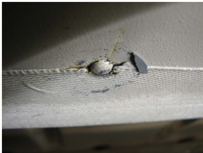
Figure 22: Dripshield fastener detail, sealant removed
