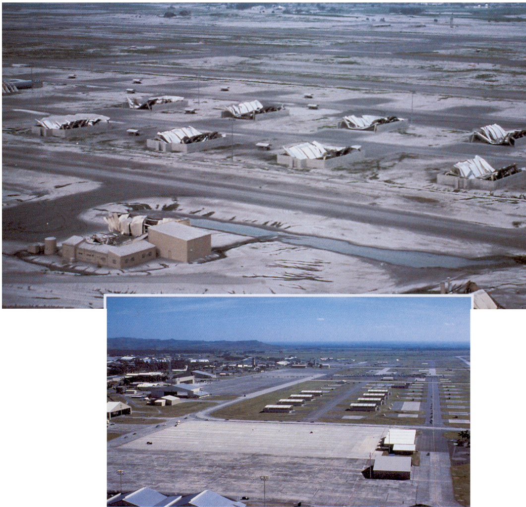
Figure 5-1. Hangars at Clark Air Force Base, Philippines, before — see insert photo (10 June 1991) — and after (24 June 1991) major eruption on 15 June, 1991. (from Casadevall)
