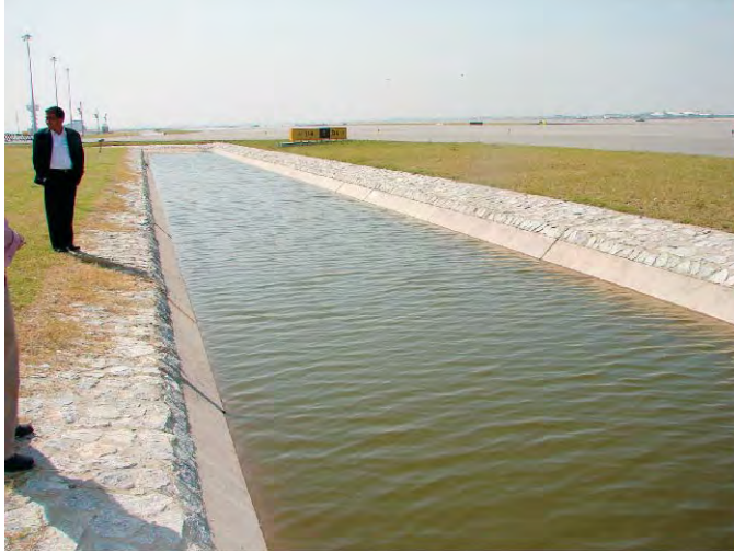
Because of the extremely high water table and frequent heavy rains in the area, it was necessary to install open canals to ensure proper drainage at this airport. The banks are cement lined and very steep to discourage wading birds. (Photo E. Cleary)
