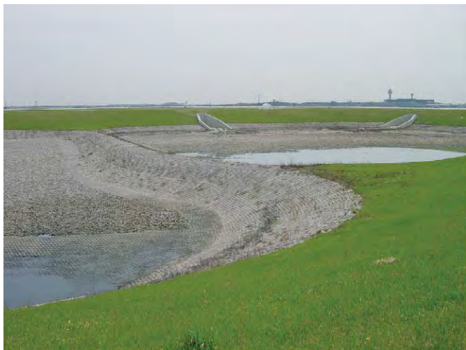
Even though this detention pond was originally designed to drain within 48 hours following the design storm, additional work is needed to ensure it drains completely. (Photo courtesy FAA)
