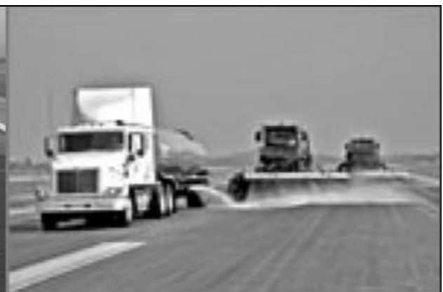
Water tanker flushing after removal followed by brooms
