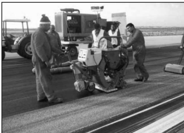
FIGURE C11 Small walk-behind shotblaster (Jenman 2006).
