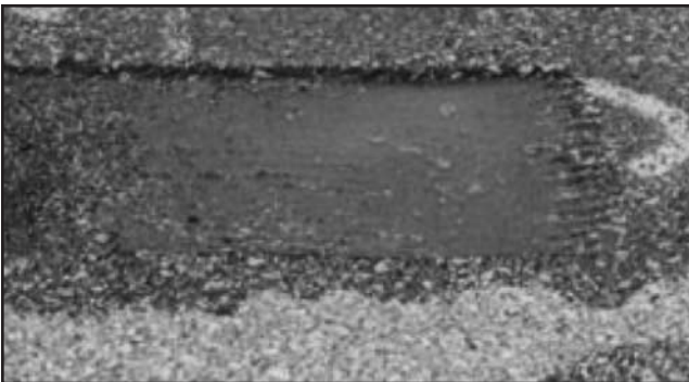
FIGURE C16 Example of grinding on asphalt surface (Skidabrader 2002).
