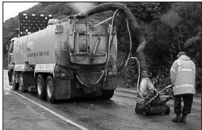
FIGURE C3 New Zealand ground-mounted and controlled watercutter (Waters 2005).
