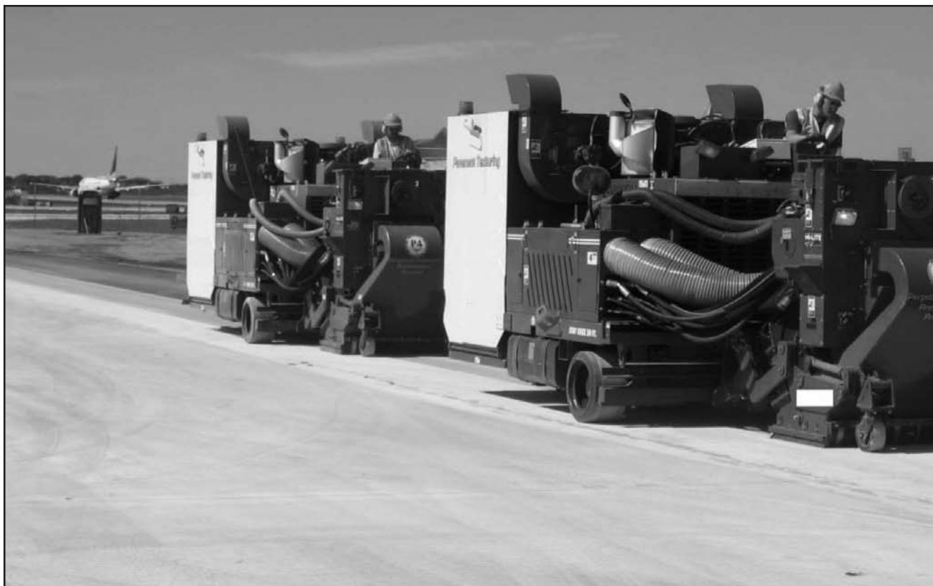
FIGURE C10 Vehicular-mounted shotblaster (Jenman 2006).
