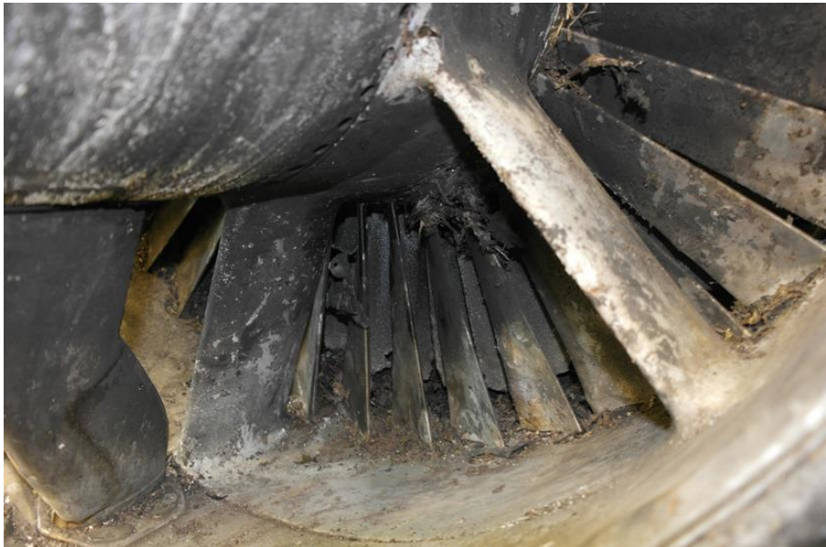
Figure 6: A closer view of the variable inlet guide vanes. The majority of debris has been removed at this stage.
