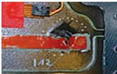
(fig.9) Resulting internal delamination
