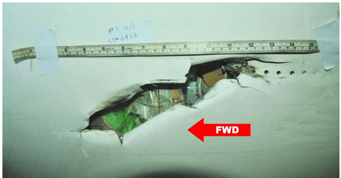
Figure 4: The hole on STA 6427
