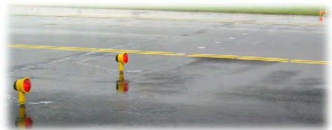
Elevated stopbar lights
