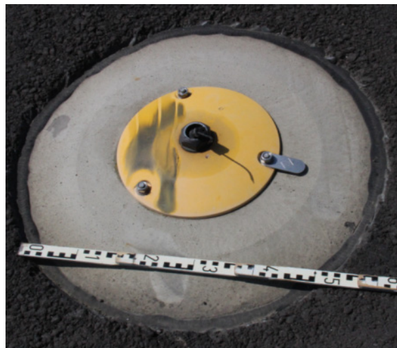
Fig. 3: Example of an overfloor lamp of the runway edge lighting, intact and torn off
