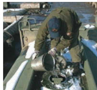
Figure 3. Improper Method to Add FSII
