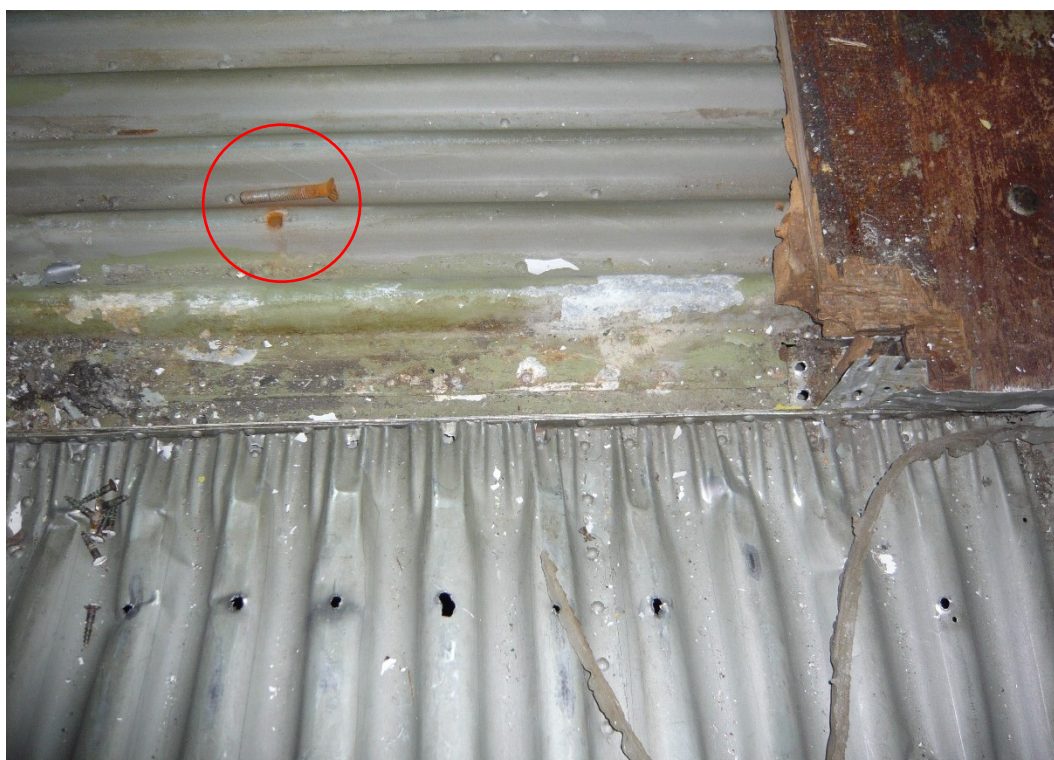
Figure 4: Close-up of figure 2 number (2) – severely corroded floor structure and bolts (red circle).
